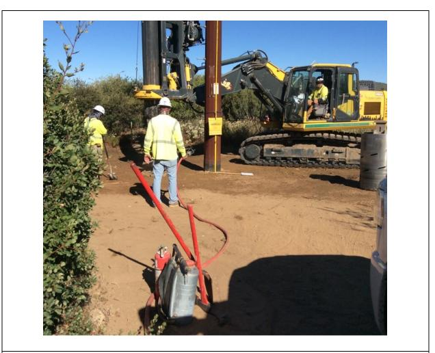
**Photo 4:** A crew was observed drilling a direct bury pole hole at P258505 (C 79B). A Dedicated Fire Patrol, at least 150 gallons of water with pump and hose, and a full set of fire tools were observed on site in accordance with the CFPPP Fire Prevention Matrix (MM FF-1) for foundation drilling on USFS land with a PAL Ev.
