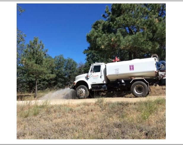
**Photo 1:** A water tender was observed applying water on Los Huecos Road (C 440 Phase II) to minimize dust emissions throughout the day in accordance with APM AIR-02.
