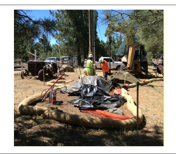
**Photo 5:** A crew was observed digging a direct bury pole hole at P45115 (C 440 Phase II). Erosion control BMPs at the site were observed in good condition in accordance with the ECP (MM HYD-1) and SWPPP (MM HYD-1, MM BIO-7).
