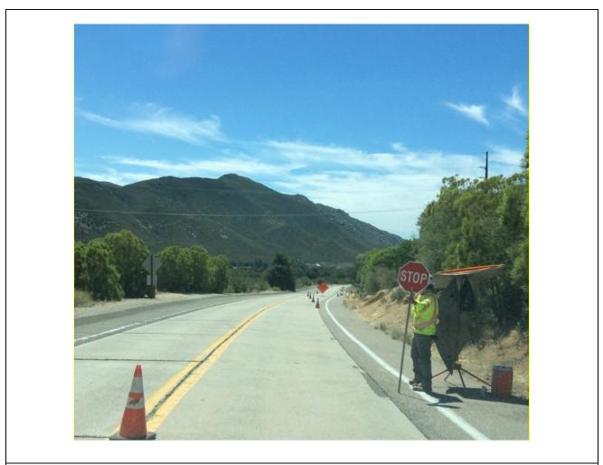
**Photo 6:** Signage, cones, flagpersons, and a clearly marked pilot vehicle were used to direct one-way traffic around the work area on Old Highway 80 (TL 629A) in accordance with the Traffic Control Plan (TCP; APM TRANS-05) and APM TRANS-02.
